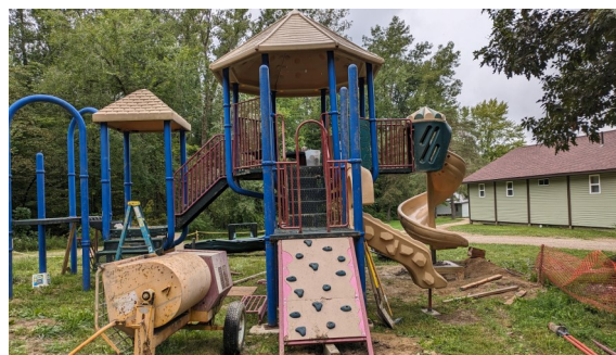
Installation of new playground area
